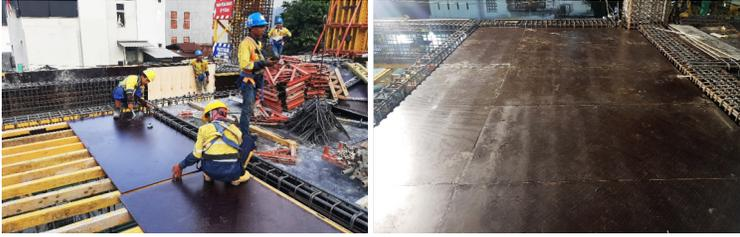
**Gambar 3.7** Panol /Papan Plywood tebal 15mm
