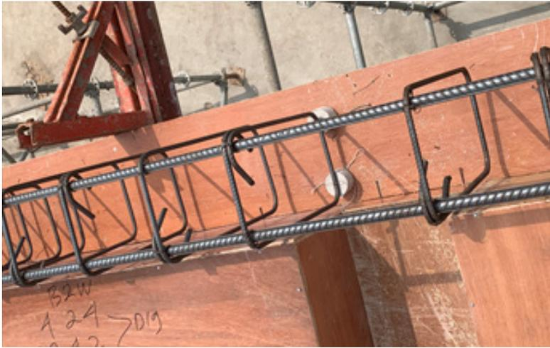
**Gambar 4.11** Beton Decking
