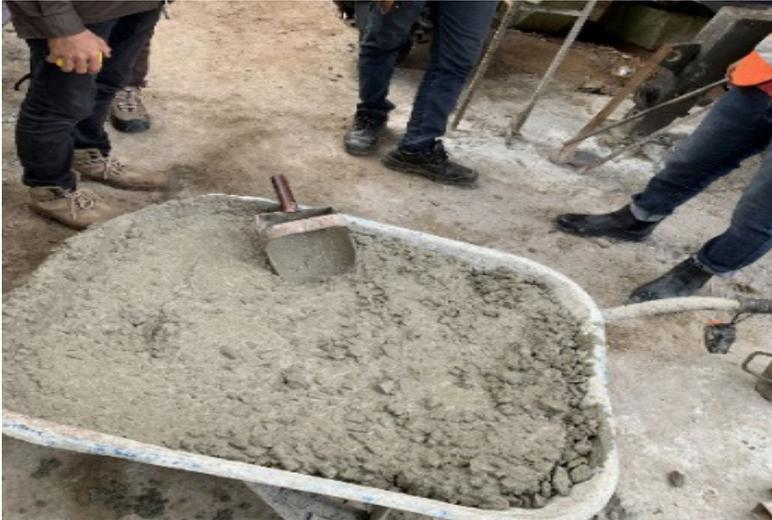
**Gambar 2.7** Beton Ready Mix
