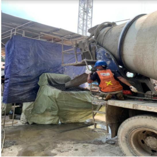
**Gambar 5.3 Distribusi Beton ke Concrete Pump**
