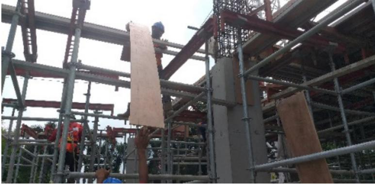
**Gambar 3.9** Meletakkan Bottomform Bekisting Diatas Suri-Suri
