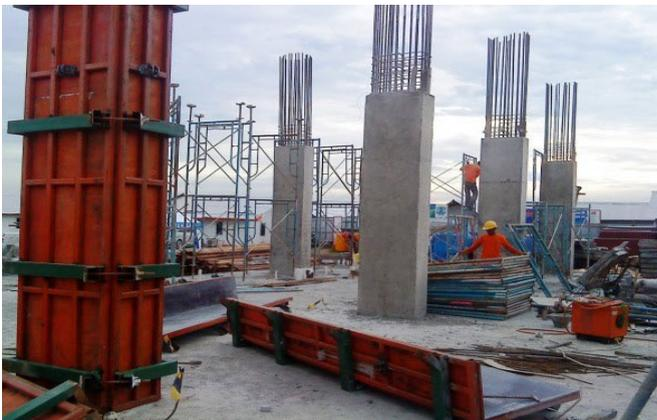
Gambar 1.2. Bekisting Semi Sistem
