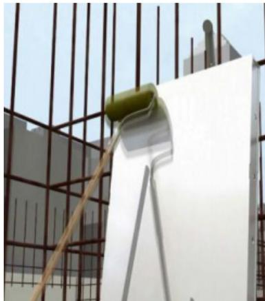
Gambar 1.22. Memasang Formwork Oil Bekisting Aluminium
