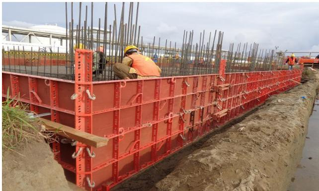
Gambar 1.3. Bekisting Sistem
