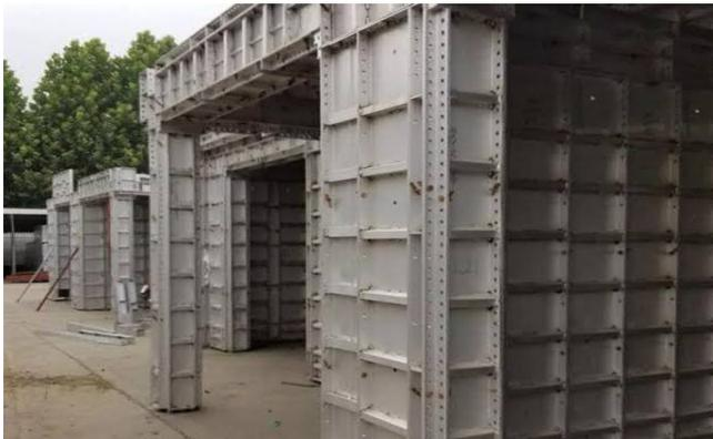
Gambar 1.5. Bekisting Aluminium
